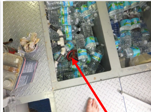
Raw Water Intake
